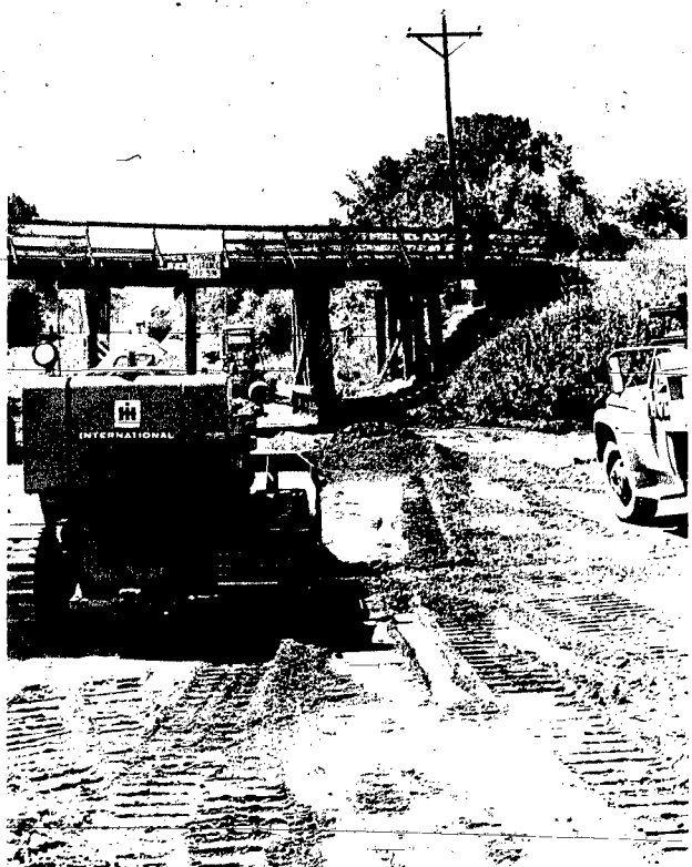
Work was progressing well Thursday on lowering of the underpass on Highway 9 on the edge of Allen. The highway had a clearance of 12 feet and five inches, but lowering of the highway will add just over another foot to that clearance, making it unnecessary for many trucks to take the detour through Allen in order to get past the underpass. This view is north of the underpass looking south.
